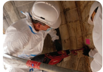
Collect of mortars from the vaults of the choir
